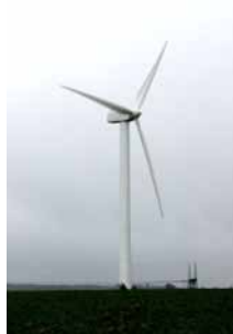
600 kW Vestas wind turbine with 47m rotor diameter
