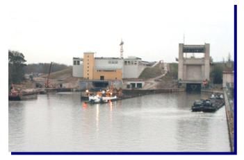
The Elbe Side Canal connects the river Elbe with the Mittelland Canal. Due to the forcast of the increase of the shipping traffic is beside the existing sluice Uelzen I a construction of a new sluice in progress. These sluice features an effective length of 190 m, a nominal width of 12,50 m and a height of stroke of 23 m. 230.000 m³ reinforced concrete were used. Therewith the sluice Uelzen II counted among to the biggest of her kind in the German domestic traffic.
